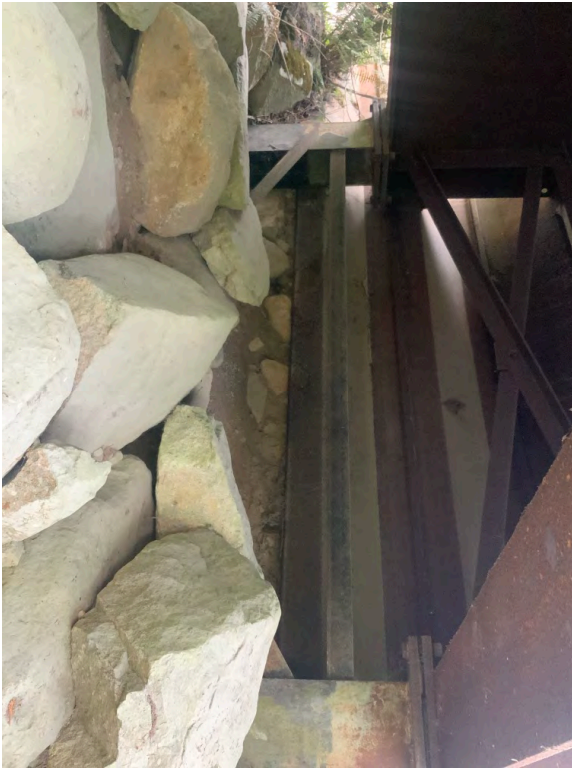
Left Bank Abutment when facing downstream
